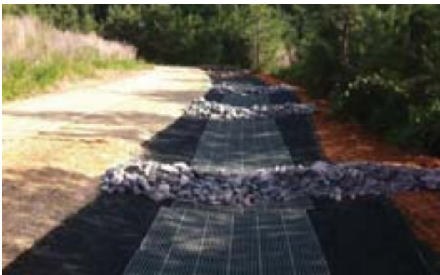
To boost performance of the VMax turf reinforcement mats in critical applications, combine with our ShoreMax® flexible transition mat to create a system that can dramatically elevate the permissible shear stress and velocity protection beyond many hard armor solutions.
